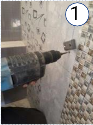
1 Mark and Drill Holes after measurement
